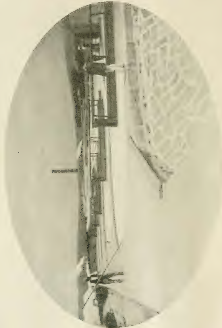
FIG. 14. CONICAL BOTTOM-DISCHARGE SETTLING PITS, THICKENING PURIFIED CLAY PULP FOR THE PIPE-LINE. (Photo, English China Clays, Ltd., St Austell)
